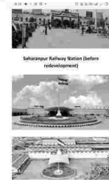
Saharanpur Railway Station (before redevelopment)
